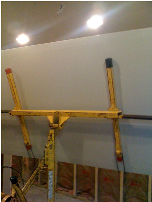
A drywall lift because Ms. Valerie has spent a lot of time in 2020 hanging drywall!
